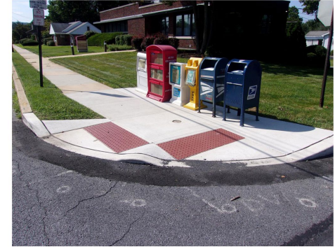
ADA Curb Ramps Kenhorst Blvd.
