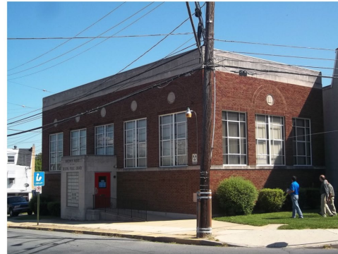
Reading Public Library Northwest Branch
